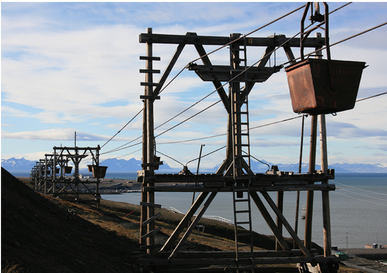
Figure 12. The iconic cable car bucks in Longyearbyen, Svalbard were originally used to transport coal from the mines to the harbour. Longyearbyen, Svalbard's largest settlement, was dominated by coal mining from around 1900 until the late 1990s. Source: Anne-Cathrine Flyen, reproduced with permission.
