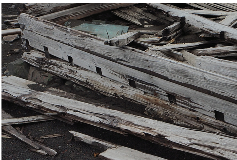
Figure 10. Detail of the remains of the magistrate's Villa in Whalers Bay on Deception Island affected by fungal decay. Source: Ann Kristin Balto, reproduced with permission.
