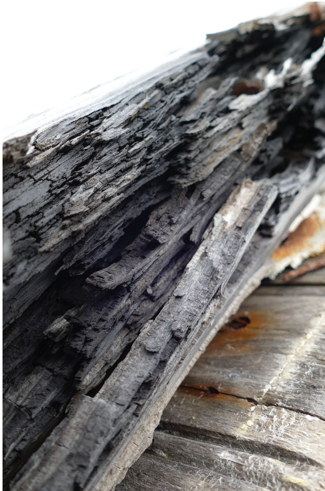
Figure 8. Detail of stranded boat in Grytviken on South Georgia affected by fungal decay. Source: Carl Erik Kilander, reproduced with permission.
