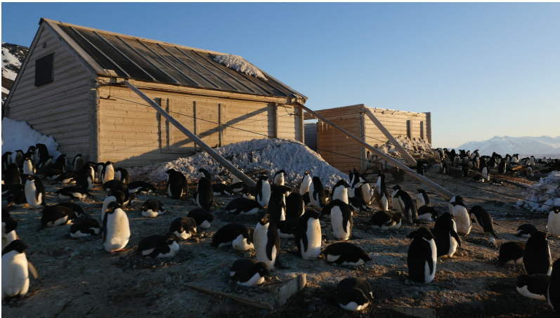
Figure 6. The Carsten Borchgrevink cabin at Camp Ridley photographed in 2016–2017. Source: Tom Edvinsen, Norwegian Broadcasting Corporation (NRK), reproduced with permission.
