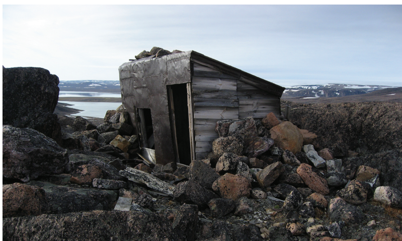
Figure 2. An emergency radio shack at Haudegen in Nordaustlandet, Svalbard. This was a manned German meteorological station built in 1944 during World War II. Source: Anne-Cathrine Flyen, reproduced with permission.
