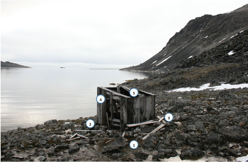
Figure 11. Microclimatic zones exemplified in-situ in a heritage trapper's cabin in Kobbefjorden, Danes Island, Spitsbergen in Svalbard: (1) Permafrost area; freezing temperatures, no free water; (2) Thawing zone; low temperature, high water content; (3) Soil contact, relative humidity (RH); moderate temperature, high water content; (4) RH, precipitation; high temperature, high water content; and (5) RH, leakages; moderate temperature, high water content. Source: Anne-Cathrine Flyen, reproduced with permission.
