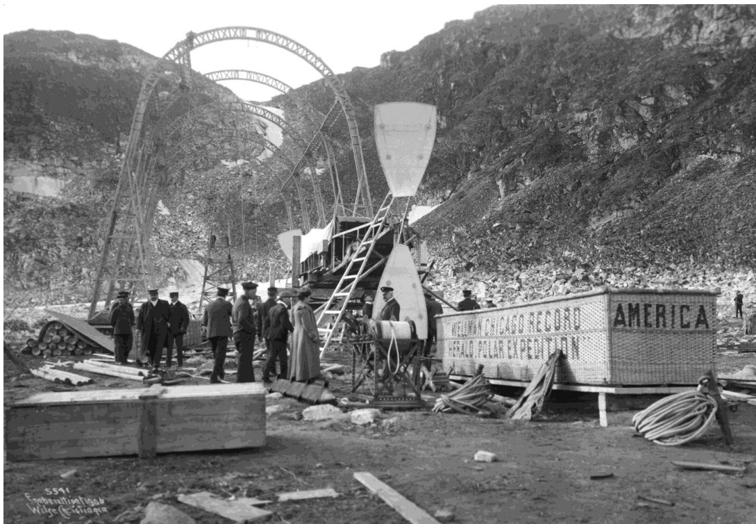
Figure 10. The airship hangar in Virgohamna showcases the pioneering work of Wellman and his crew in the field of airship technology. The photograph taken in September 1906 captures the presence of engines, the hangar, and a basket gondola attached beneath the airship, providing space for the crew and machinery. Photo: Wilse, A.B./Norsk Folkemuseum [63].
