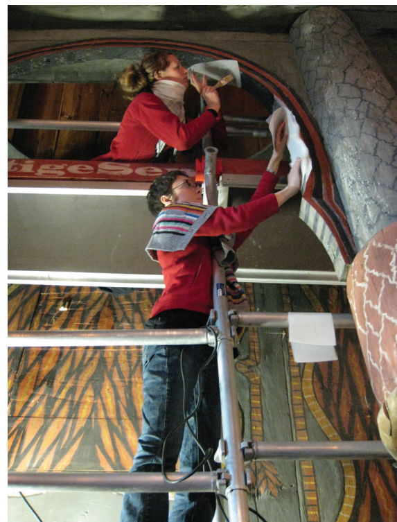
Figure 3. Consolidating distemper decorative painting with sturgeon glue in Ringebu stave church. Photo: Anne Apalnes Ørnhøi, NIKU, 2010.
