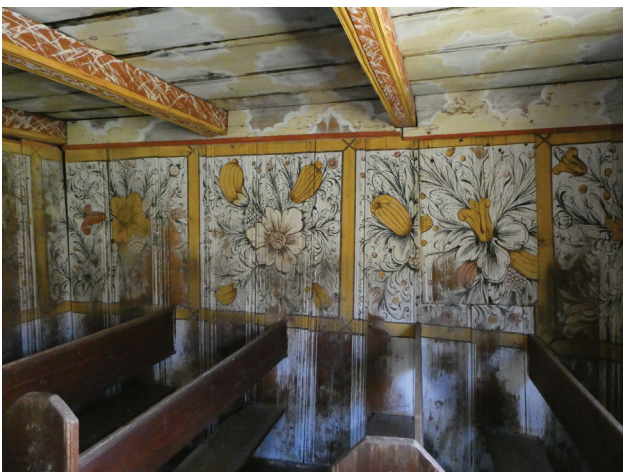
Figure 1. Example of distemper decorative painting in Nore stave church. Photo: Nina Kjølseth Jernæs, NIKU, 2020.
