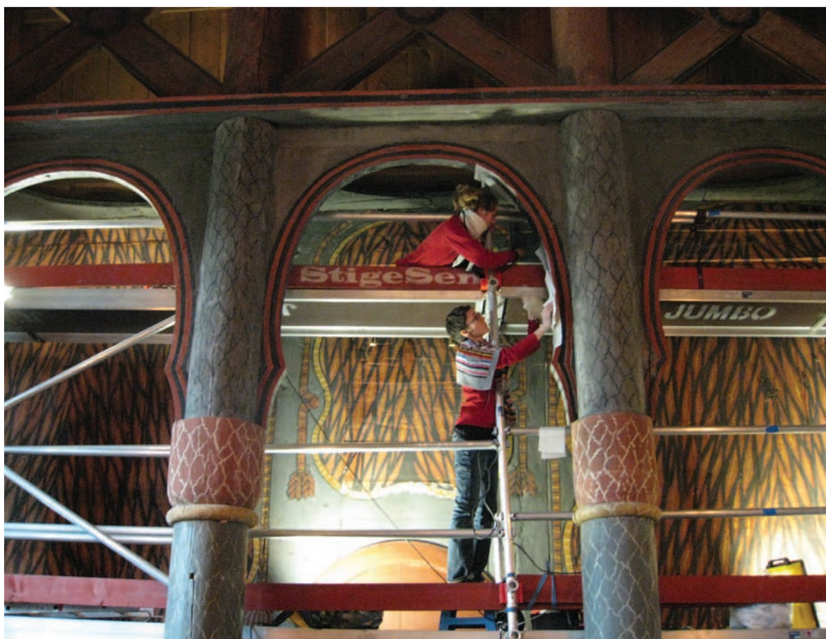
Fig. 3. Consolidation of distemper paint in Ringebu stave church. (Photo: Anne Apalnes Ørnhøi, NIKU, 2010.)
