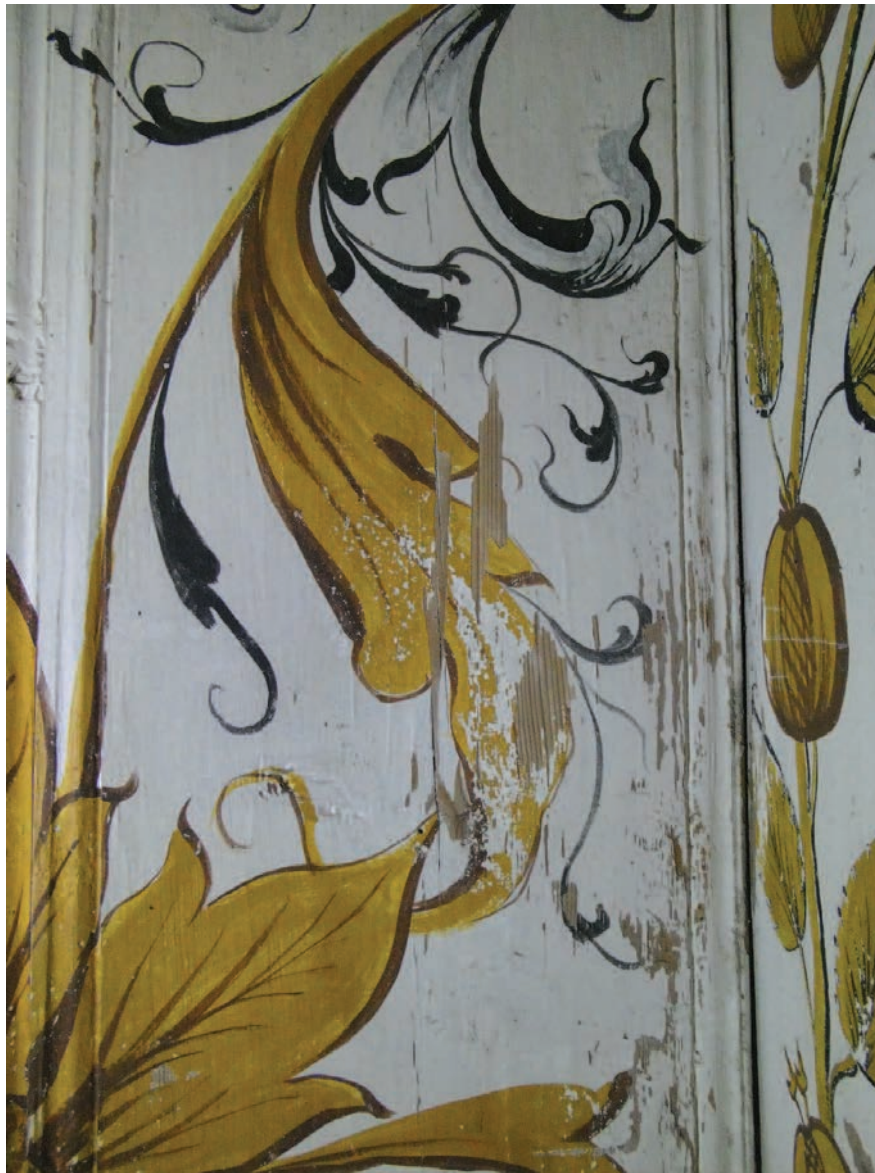
Fig. 2. Monitored area in Nore stave church where flaking paint has recurred multiple times after being consolidated. (Photo: Nina Kjølsten Jernæs, NIKU, 2020.)
