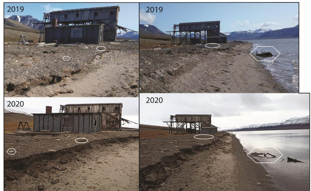
Figure 4. Comparison of shoreline position and morphology between 2019 and 2020 around some of the most important cultural heritage buildings and remnants along the sea in Sector 1 (no. 4 and no. 7). White ellipse and hexagons represent identical objects in the respective photographs.
