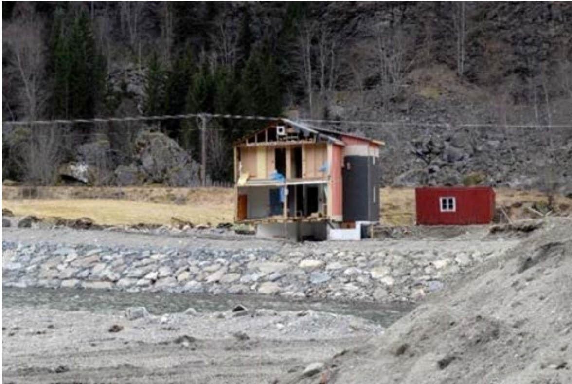
Image 3 Securing the riverbank after the flood. In the background is one of the houses that were destroyed by the ravages of the water. Photo: Marte Boro, Riksantikvaren
