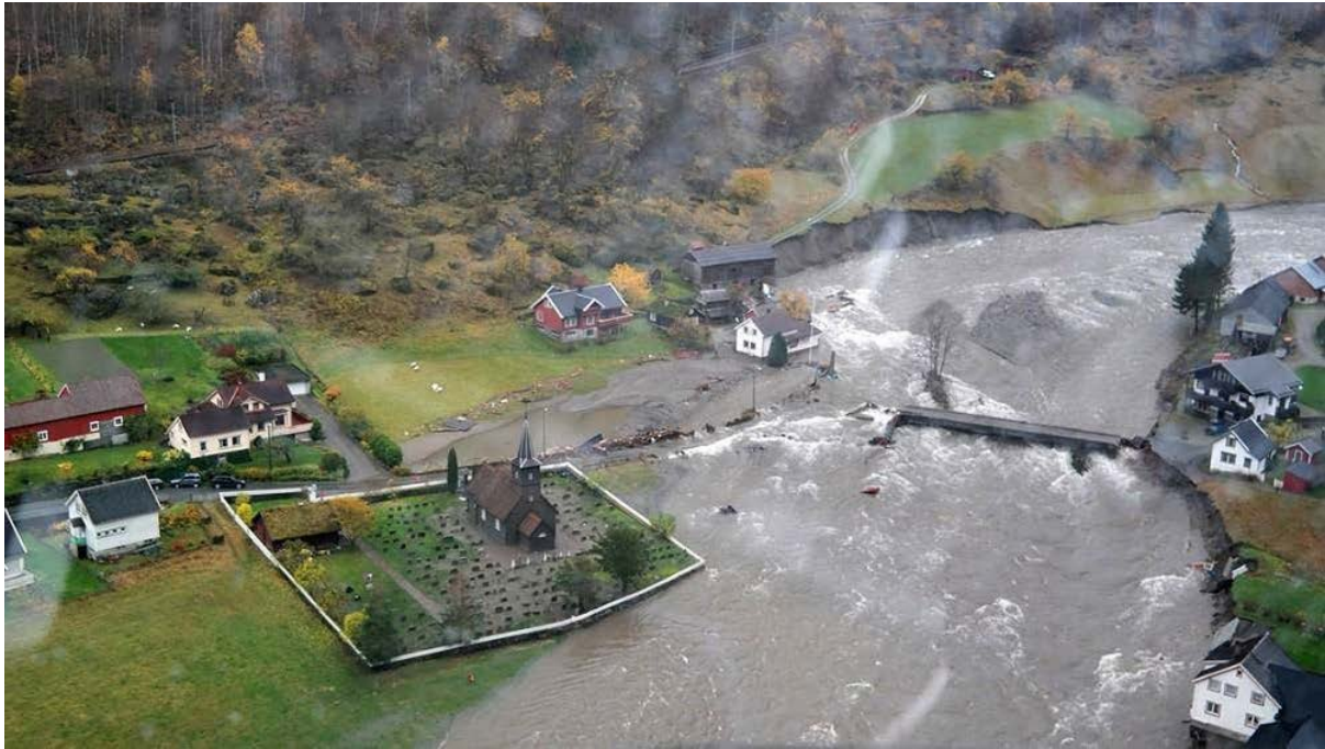
Image 5 Flood 2014. Several buildings, land and roads were washed away by the flood. Flåm church and the graveyard after the top flood tide. Photo: Oddleif Løset, NRK
