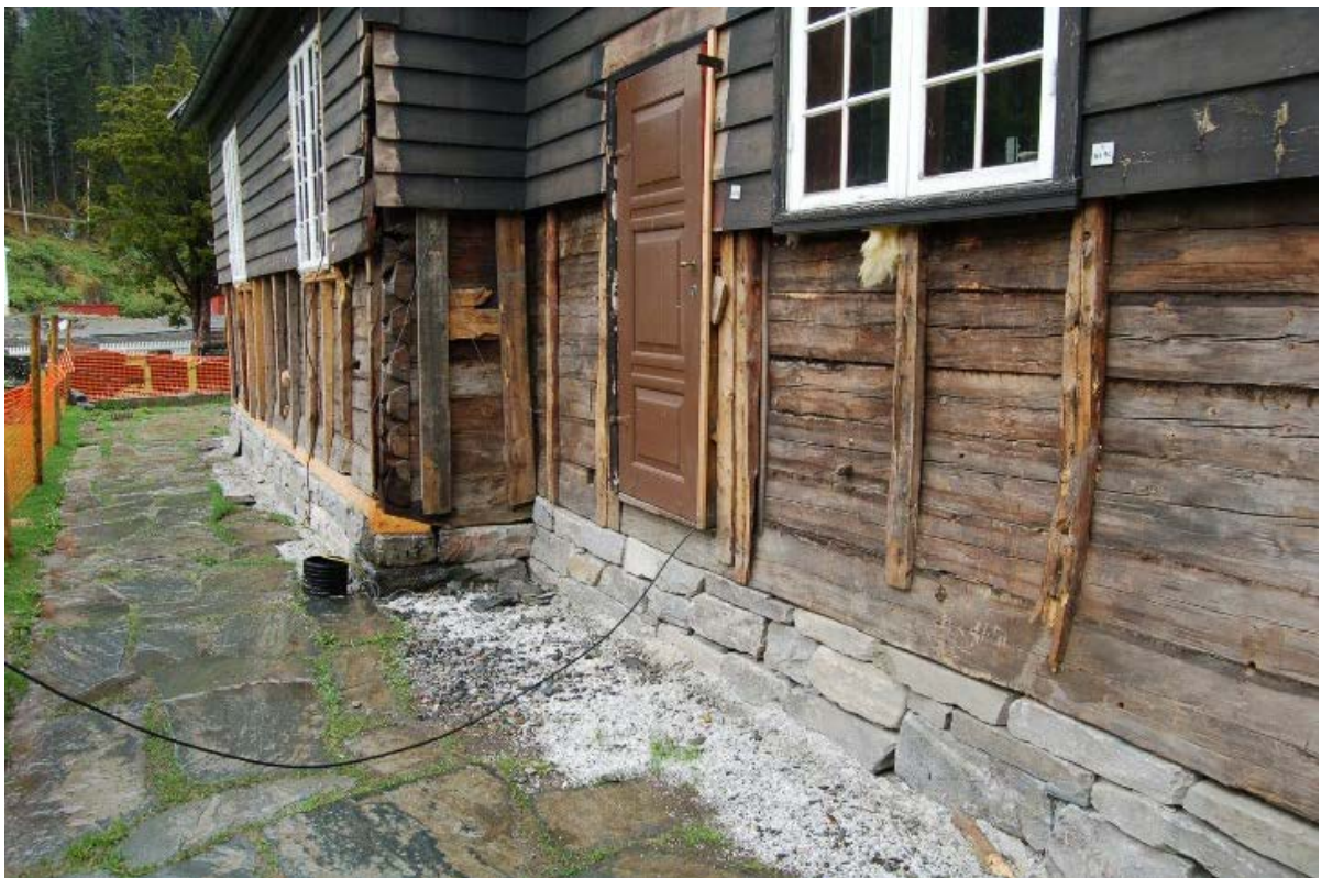
Image 8 Finalising the raise of the building. Photo: Kjersti Ellewssen, Riksantikvaren
