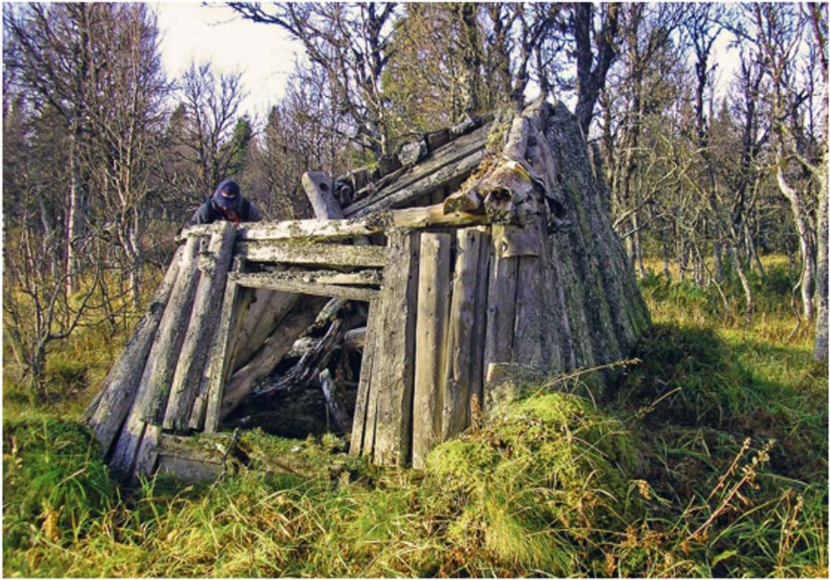
Image 21 The camp's traditional tipi, made from turf and wood, falling into disuse and deteriorating quicker. Photo: Jerker Bexelius, Stiftelsen Gaaltije
