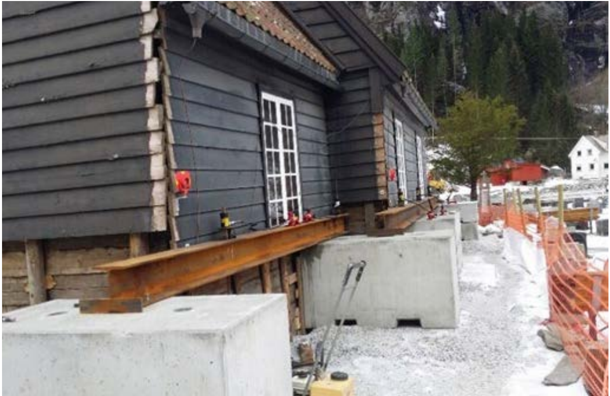
Image 7 Work in progress. Photo: Monica Finden, Aurland commune
