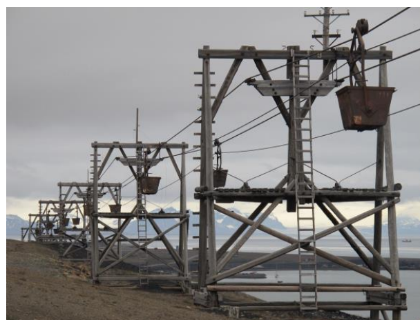
Fig. 5. Wooden structures with high risk of fungal decay where the wooden pylons are in contact with soil. Photo: Mycoteam/J. Mattsson
