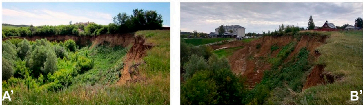
Figure 4. Views on the landslide at site 2 in 2003 ((A)—front view, (A')—lateral view) and in 2019 ((B)—front view, (B')—lateral view).
