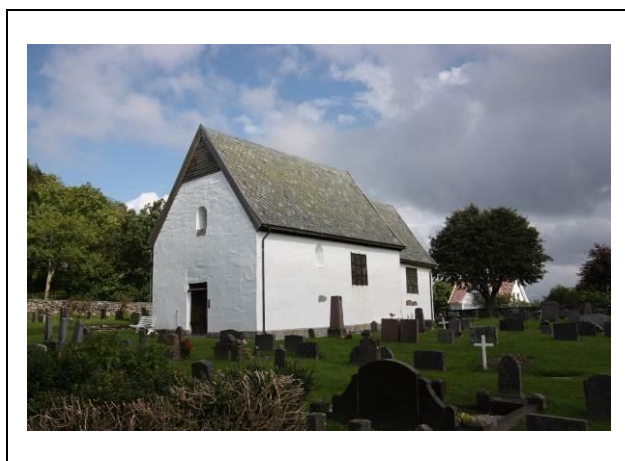
Figure 1. Moster Old church viewed from the south-west. It is a typical Norwegian building in Romanesque style with a rectangular nave and a small chancel with saddle roof.
