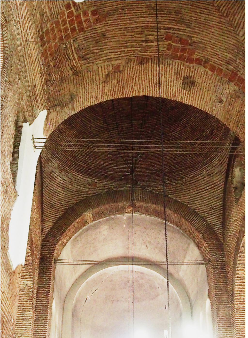
Indoor wall strengthening implementations in the St. Sofia Basilica. PHOTO: NIKU
