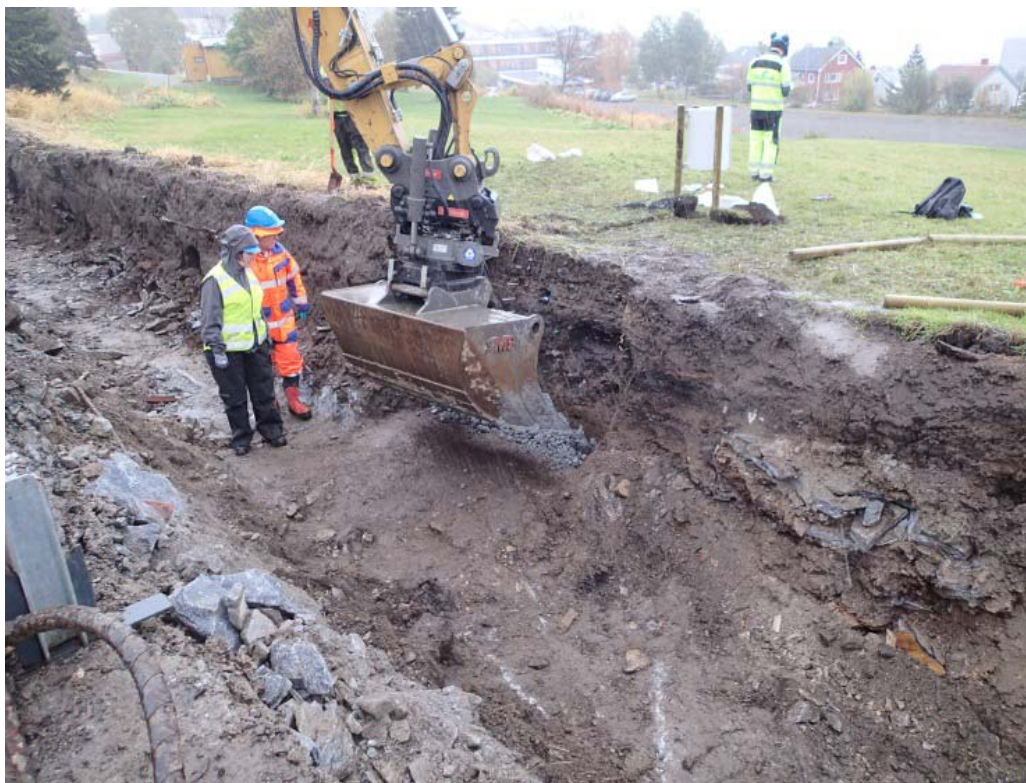
Figure 13 Securing of section at Saurbekken with clay #1, lifted by the digger. Photo: MVH Consult.
