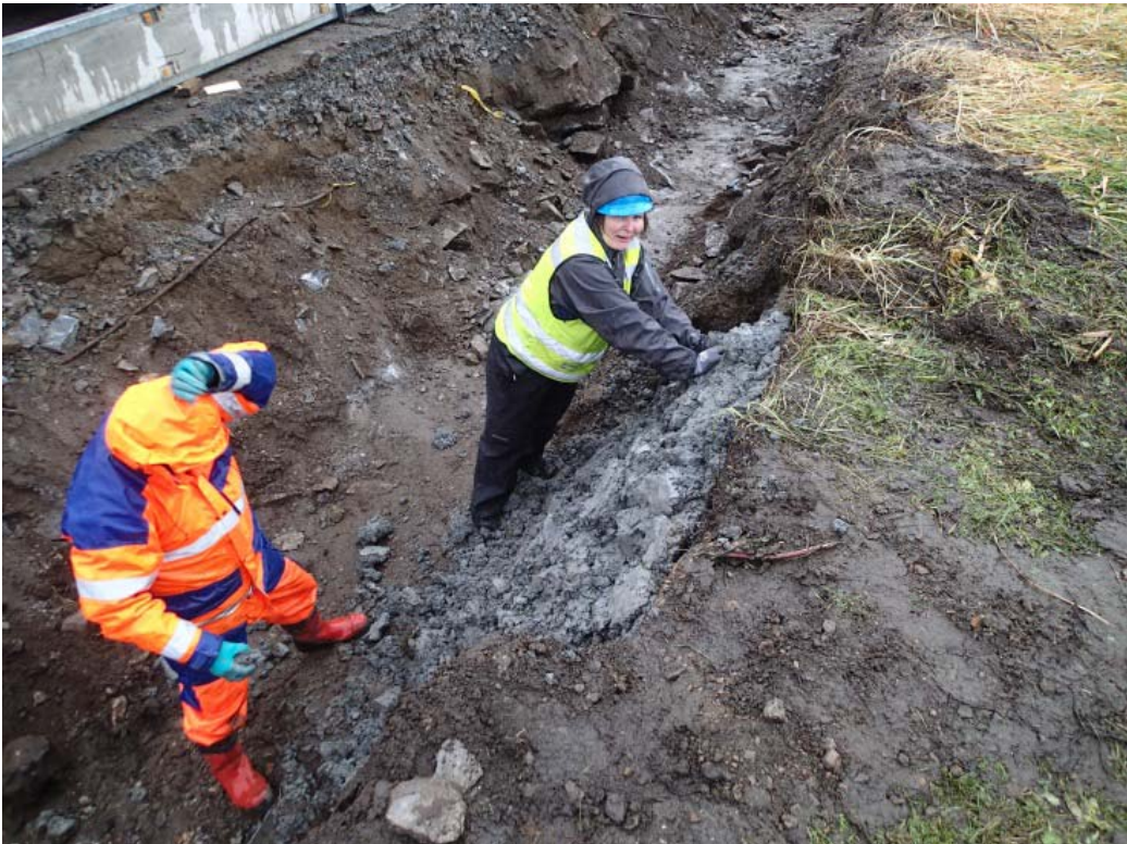
Figure 15 Securing of section at Saurbekken with clay #3. Photo: MVH Consult.
