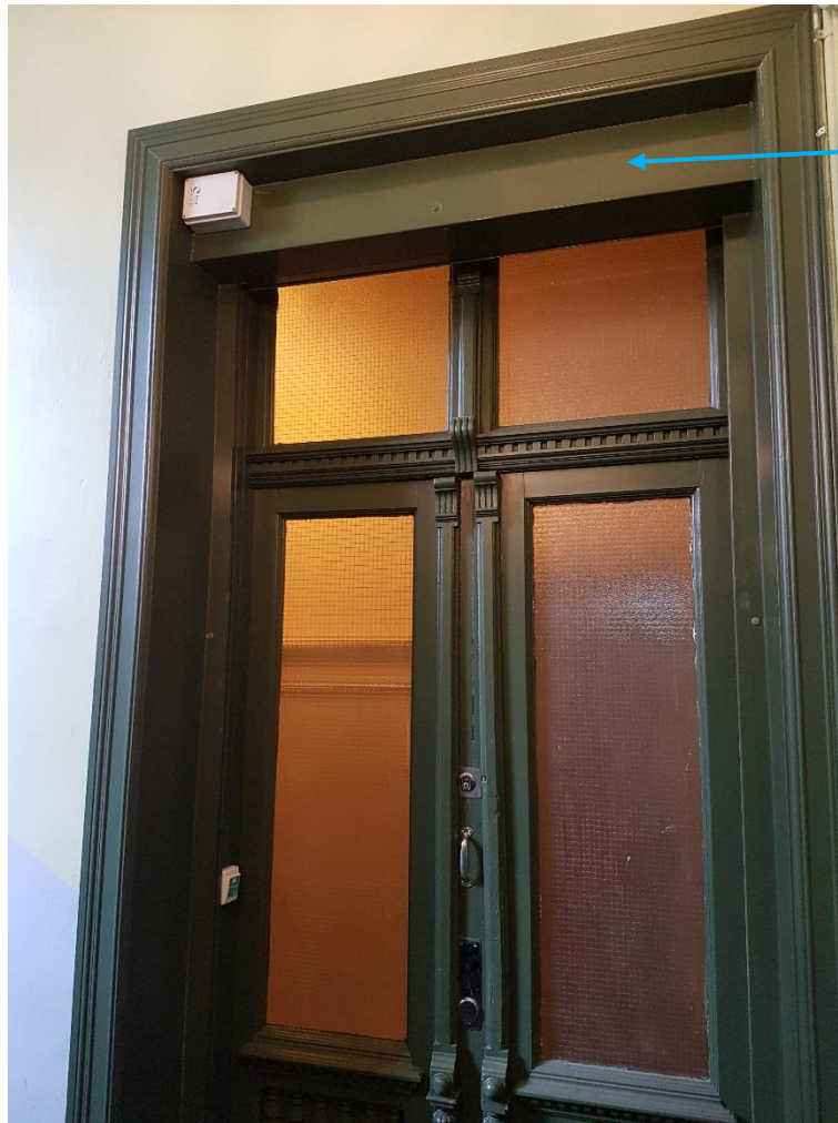
Figure 2-4 Fire curtains in front of stairwell door, Oslo. The fire curtain is inside the horizontal green box on the upper part of the door, see blue arrow. Photo: A. Korsaksel, Byantikvaren, 2018.
