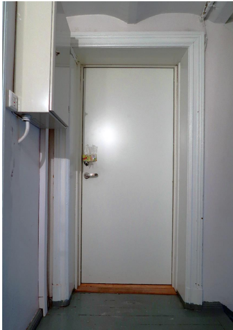
Figure 2-1 An example of replacement of unknown original door by a simple fire-rated door. Photo: B. Wedvik, NIKU, 2017.
