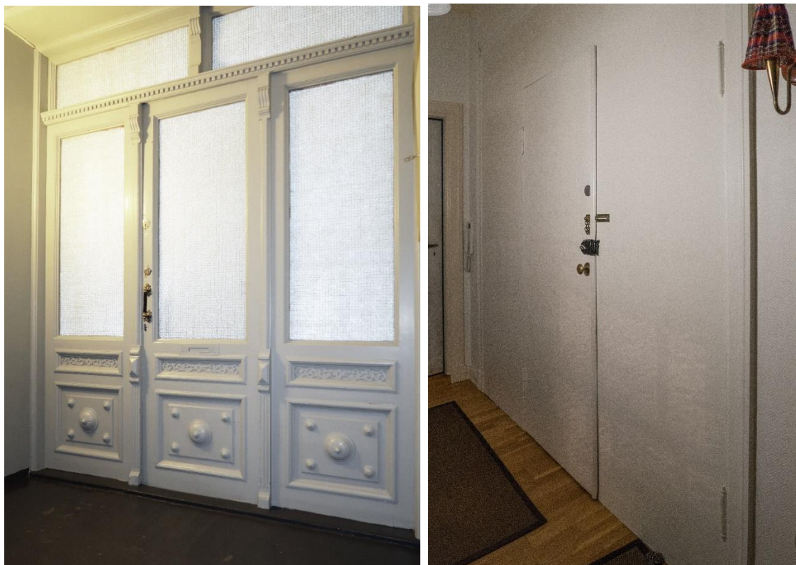
Figure 2-2 The picture to the left shows an example of door upgrading following The SINTEF Building Detail Sheet 734.503, stairwell side. The picture to the right is an example of door upgrading following The SINTEF Building Detail Sheet 734.503, apartment side. Photo: B. Wedvik NIKU, 2017.
