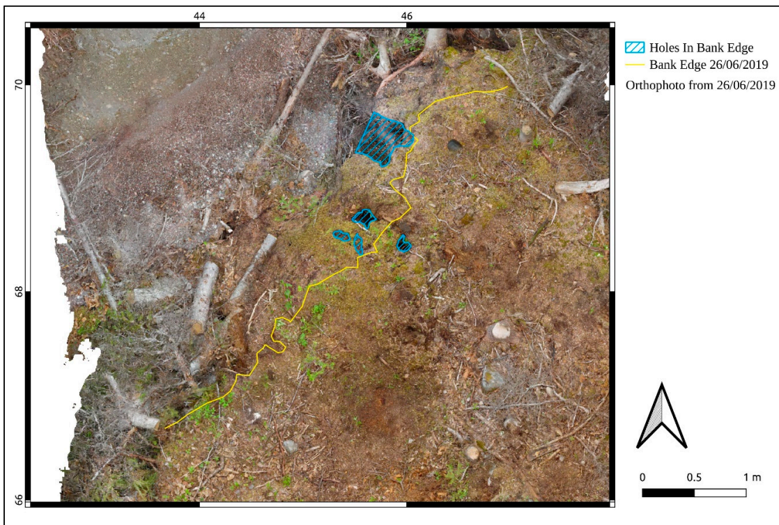
Figure 9. Holes that began appearing in the bank on 26/06/2019.
