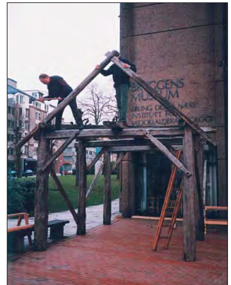
In connection with the seminar in 1998, the skeleton of a trestle-frame building was raised outside Bryggens Museum.
