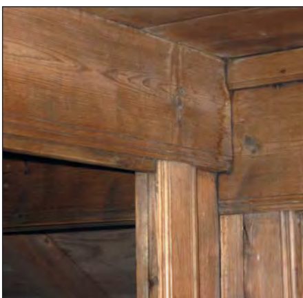
Figure 10. Decorative mouldings on beams and posts in the glasstova of the house from Múli.
