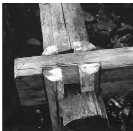
Figure 11. Corner-joint (of head beams and post) in an old house in Mi(d)vágur, photoed by Sverri Dahl 1952 when the house was under repair.
