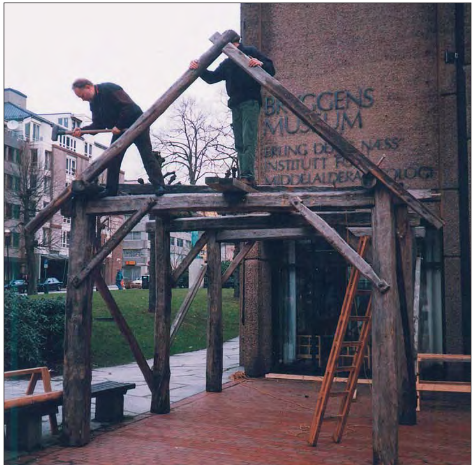
The construction of the trestle-frame building that was raised outside Bryggens Museum as a part of the seminar.
