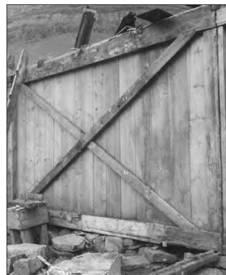
Figure 8 (Right). «St. Andrew's cross» supporting the constructive framework of the house from Múli. Photo from the removal 1961.
