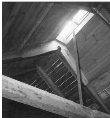
Figure 3. The louvre in the roof is the only source of light in the roykstova of the house from Múli.
