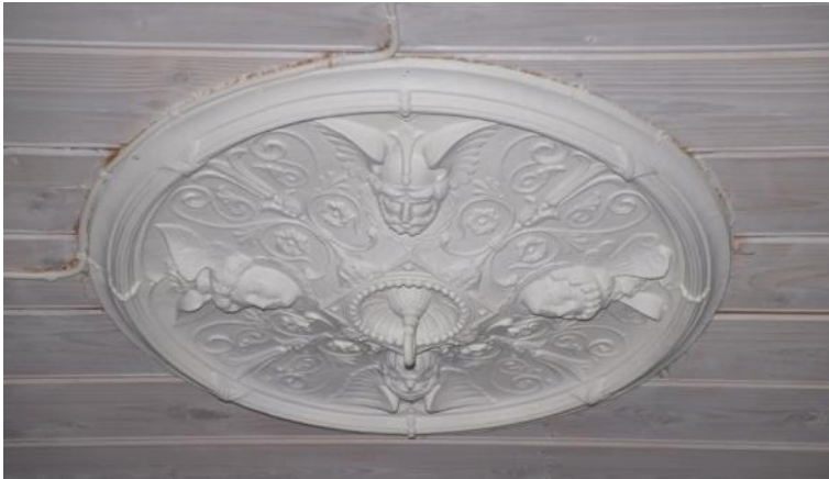
Gipsrosett i himling
