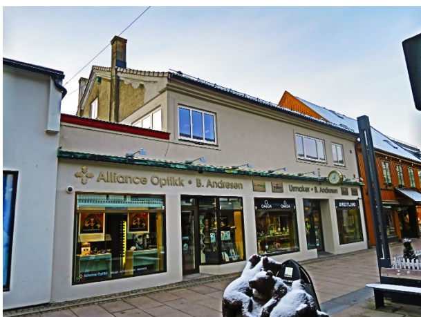
Figur 3-15 Dronningens gate 8 (NIKU 2018).
