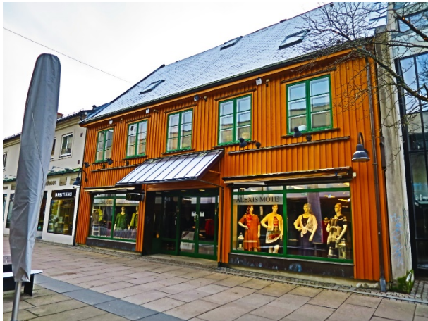
Figur 3-16 Dronningens gate 10 (NIKU 2018).
