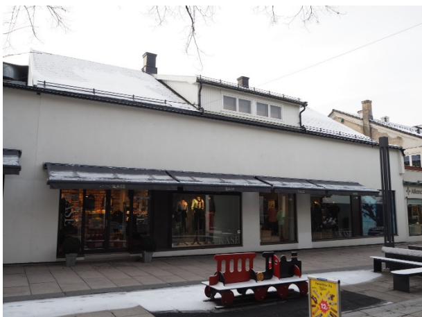
Figur 3-14 Dronningens gate 6 (NIKU 2018).
