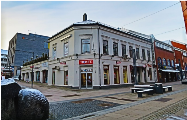
Figur 3-18 Dronningens gate 14 (NIKU 2018).
