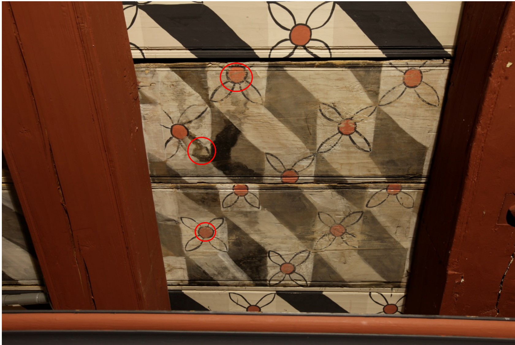
Figur 6 Felt 2, løs maling markert.
