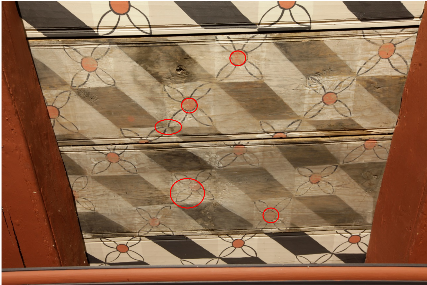
Figur 8 Felt 4, løs maling markert.
