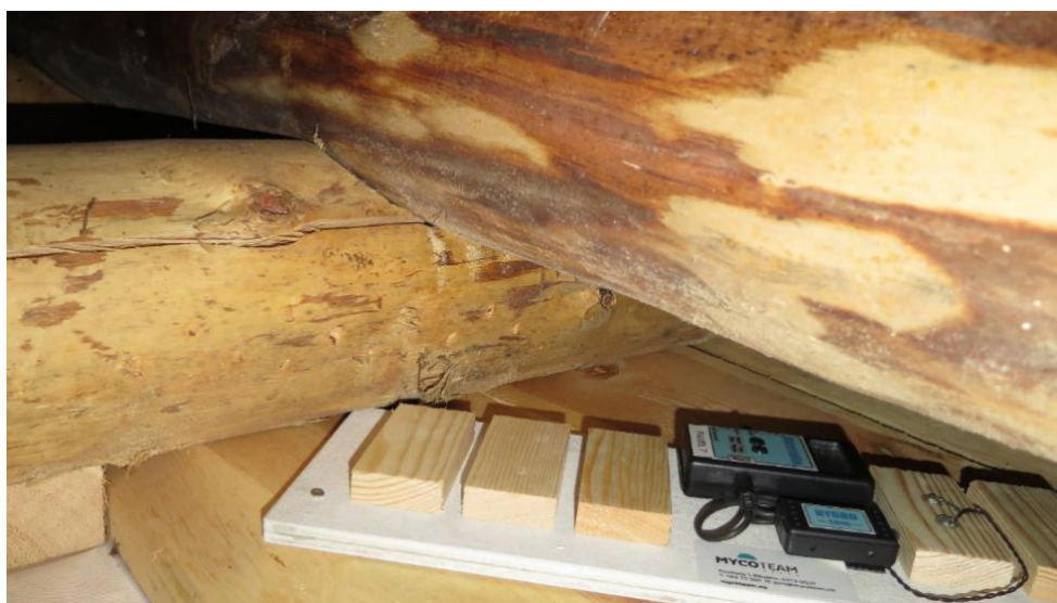
Figure 3. Climate panel. Photo: NIKU.
