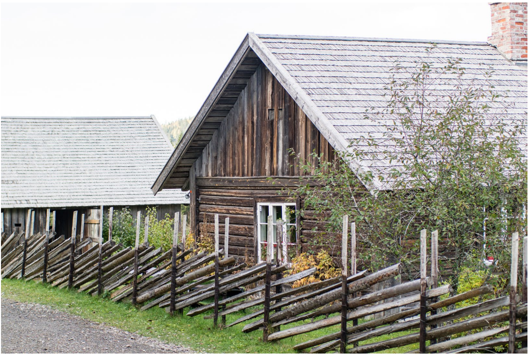
Figure 1. The Prøysen cottage (Prøysenstua) today. Photo: Jan Löfgren.
