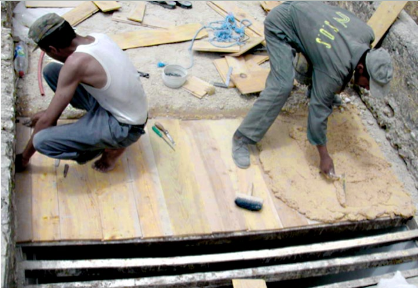
Roof structure under rehabilitation ©
