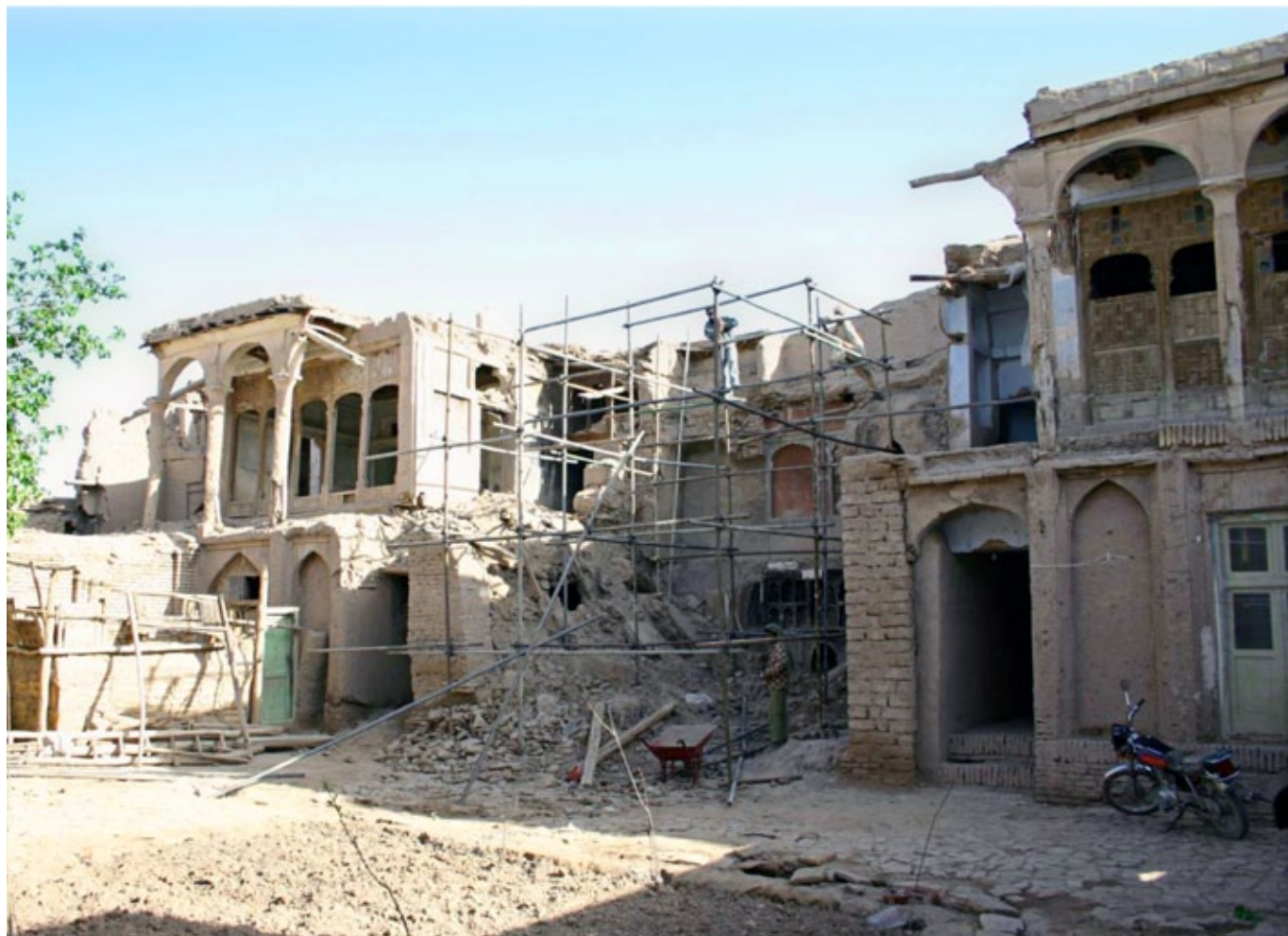
Attarbashi house in Herat old city before conservation ©
