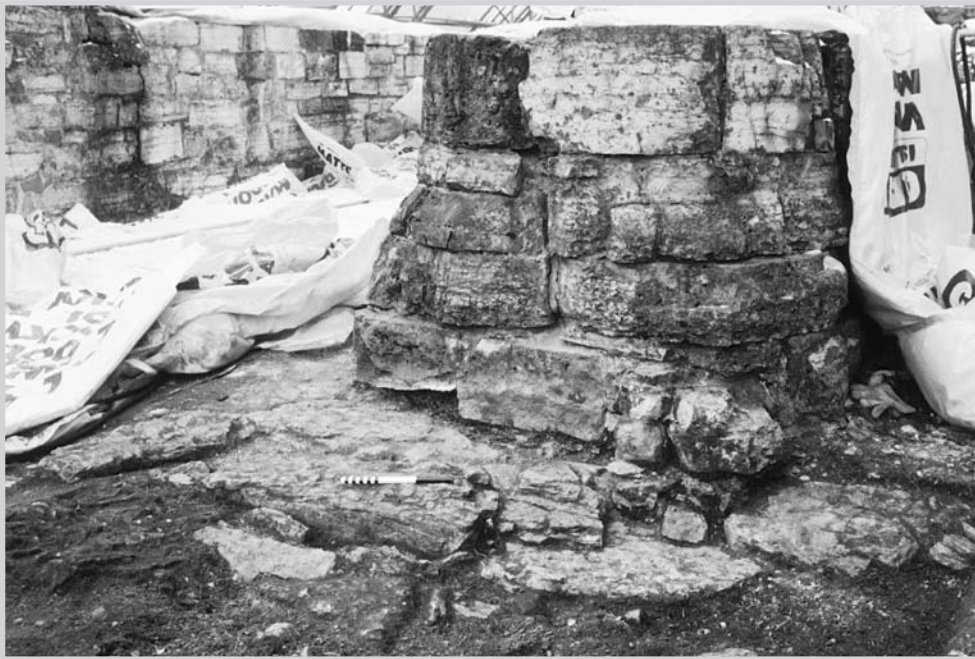
Fig. 39. Foundation R108, group 2:7 beneath and west of column base R111. Photo Bruce Sampson, NIKU.
